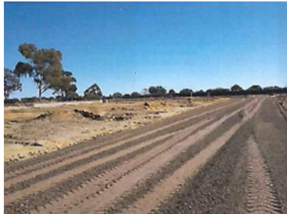
Recycled road-base, The Amble Estate. (Image supplied by Porter Consulting Engineers)
