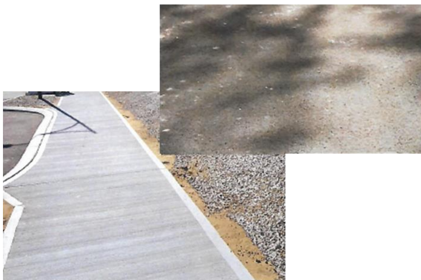
Path and pavement incorporated recycled product – concrete, sand, and asphalt. The Amble Estate (Images supplied by Porter Consulting Engineers)
