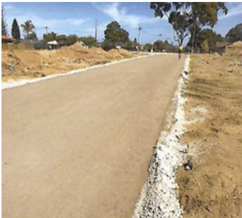
Recycled road-base, The Amble Estate. (Image supplied by Porter Consulting Engineers)
